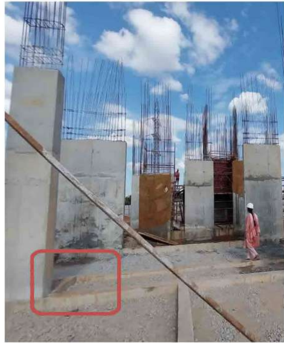
Error in termination of the top bar.
