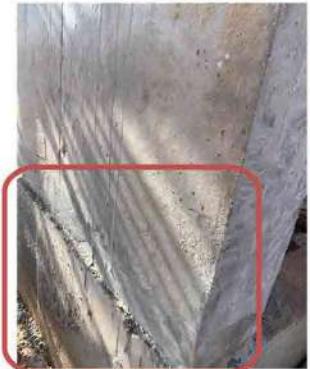
Mis-alignment of Plinth beam and column, Extension from alignment bulge in the plinth beam.
