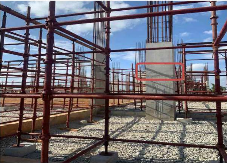
honeycomb issue and area has been plastered
