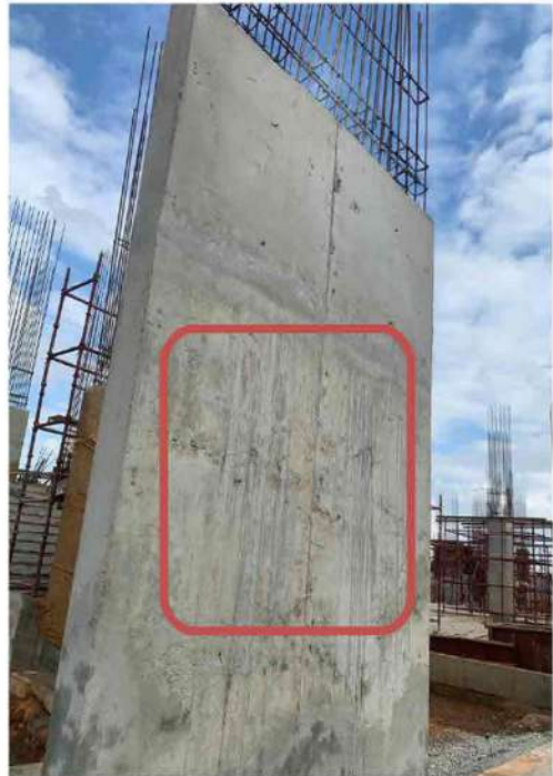
Double shuttering : Mis-alignment at the centre
