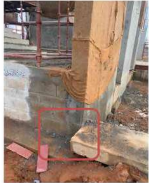
Mis-alignment of Plinth beam and column, Extension from alignment bulge in the plinth beam.
