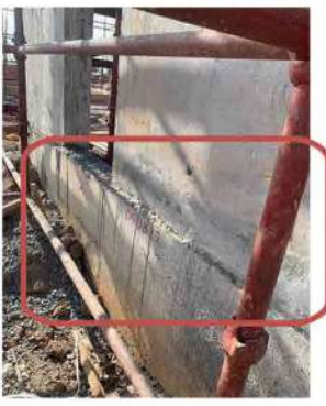
Mis-alignment of Plinth beam and column, Extension from alignment bulge in the plinth beam.
