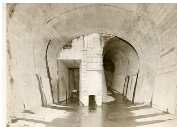
Catskills Aqueduct Headworks, Built 1907-1915
